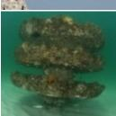
Concrete Disk Reef: 8 ft. tall, three or more rock or shell embedded concrete layers mounted on a piling. These particular reefs will be deployed within 500 ft. from shore making them easily accessible. An <a href="underwater camera">underwater camera</a> was recently installed at a similar site offshore of Navarre Beach.
