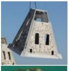
**Small Tetrahedron Reef**: 6-8 ft. tall, 10-ton hollow concrete walled structure with three or more sides. This structure is the most common artificial reef structure in the region.
