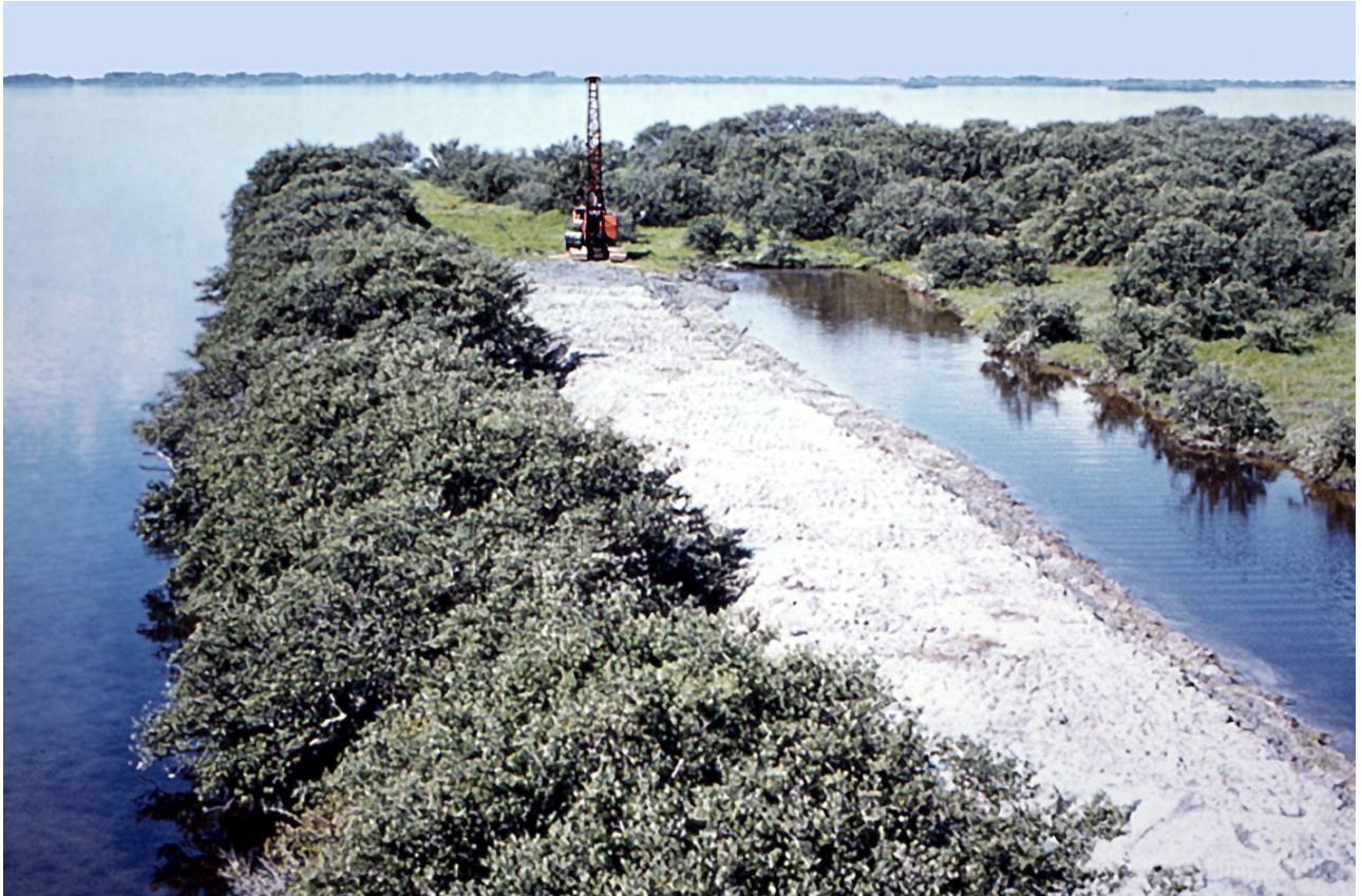
Figure 12.4. Construction of the last impoundment along the IRL in 1974 for the control of salt marsh mosquitoes using the typical dragline excavator. The Gumbo Limbo Island impoundment was the first and only impoundment along the IRL built purposefully for rotational impoundment management. Photo courtesy of the Florida Medical Entomology Laboratory Archives.
