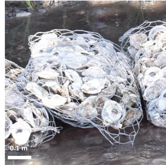
Galvanized metal gabions
