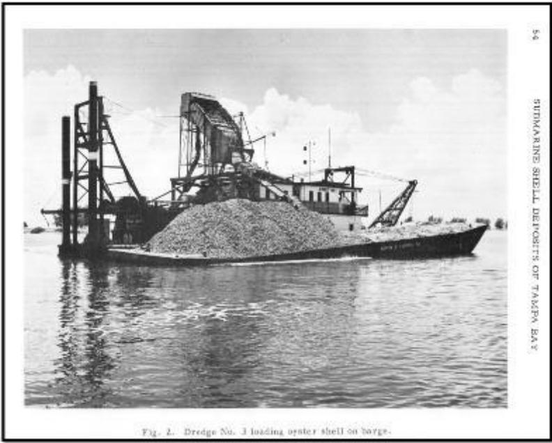
Fig. 2. Dredge No. 3 loading oyster shell on barge.
