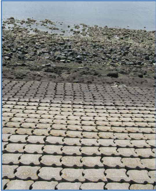
Defenses along Netherland's dikes tiles above, asphalt below
