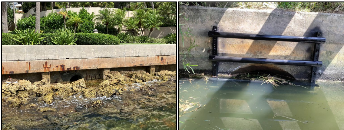
Photo of culvert and living shoreline at Brickell Key in Biscayne Bay, Miami-Dade County (left). Photo of grated culvert in Cape Canaveral, Brevard County (right).
